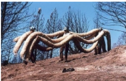
Carrying Straw Wattles
